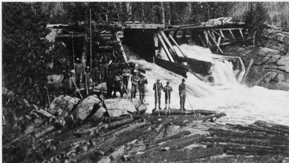
Plate 4. Logging Dam on the Little Wolf River, Waupaca County, 1890's. (Courtesy Oshkosh Public Museum, Oshkosh, Wisc.)
