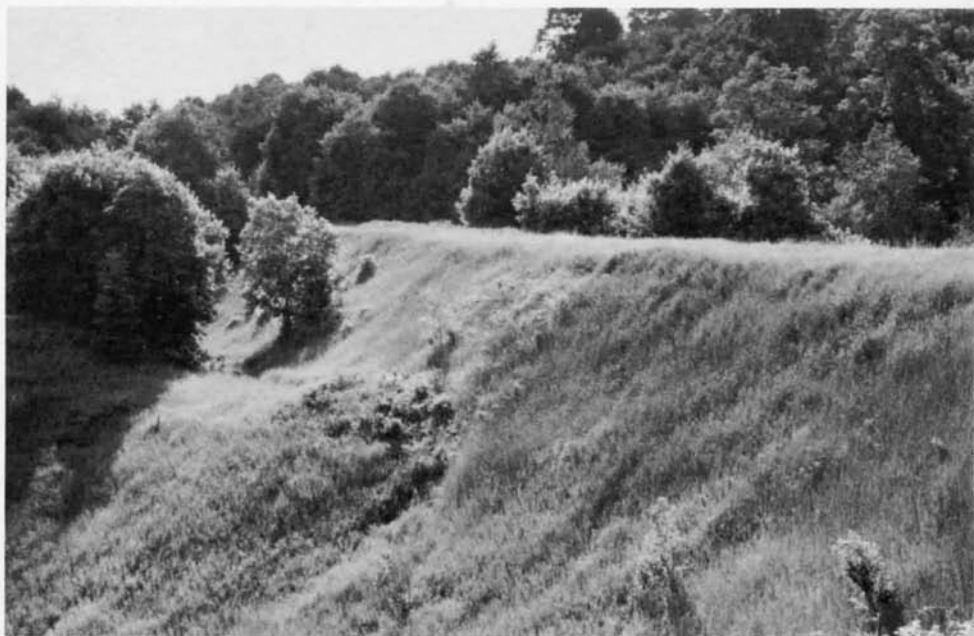
Plate 16. Fill thirty-two feet high and several hundred feet long near Butternut Lake on the Thunder-Lake Narrow Gauge. (1960, Courtesy Harry Huston.)
