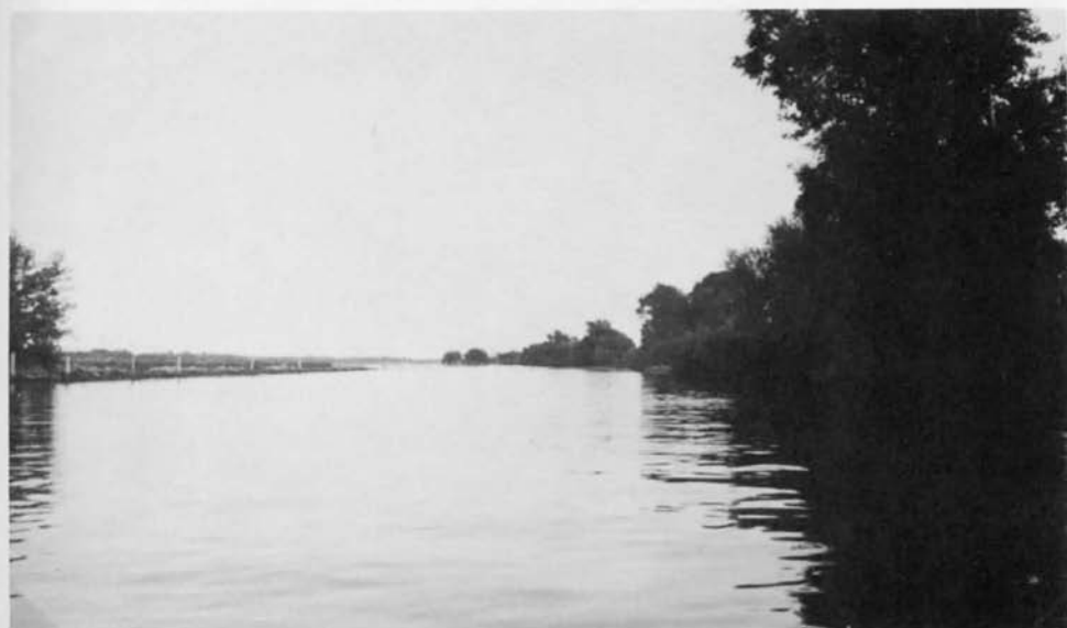
Plate 8. The Boom Cut constructed to give Boom Bay direct access to the Wolf River. (Author, 1970.)
